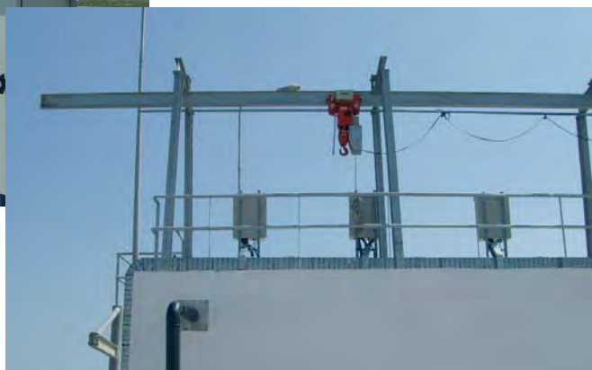
Electric Chain Hoist with electric trolley Type 66/04 AKE capacity: 5 t installed in a sewage plant in Tunisia
