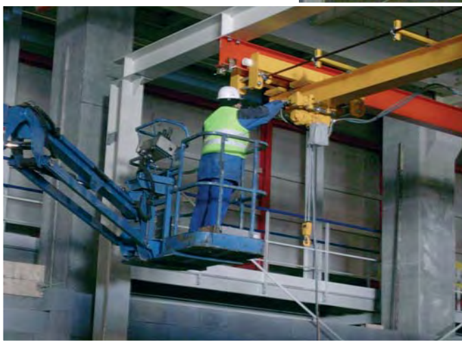
crane installation
